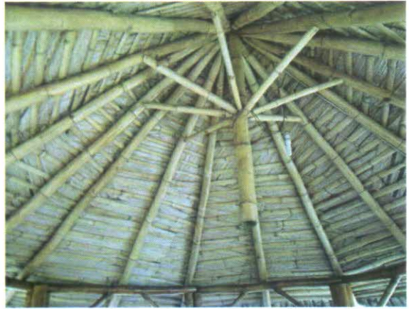
Plate 4.4: A roof truss made from bamboo
